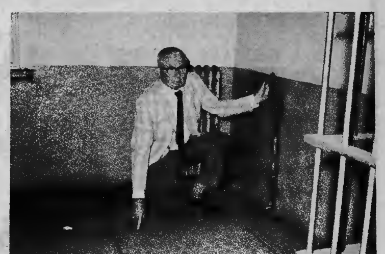
BUILT-IN GALLOWS — Sheriff Wimberly indicates the lever (at right) and the line of the trapdoor inset in upstairs corridor of old jail, a grisly relic of long-ago days when counties handled their own executions.—(Photo by V. Nicholson)
