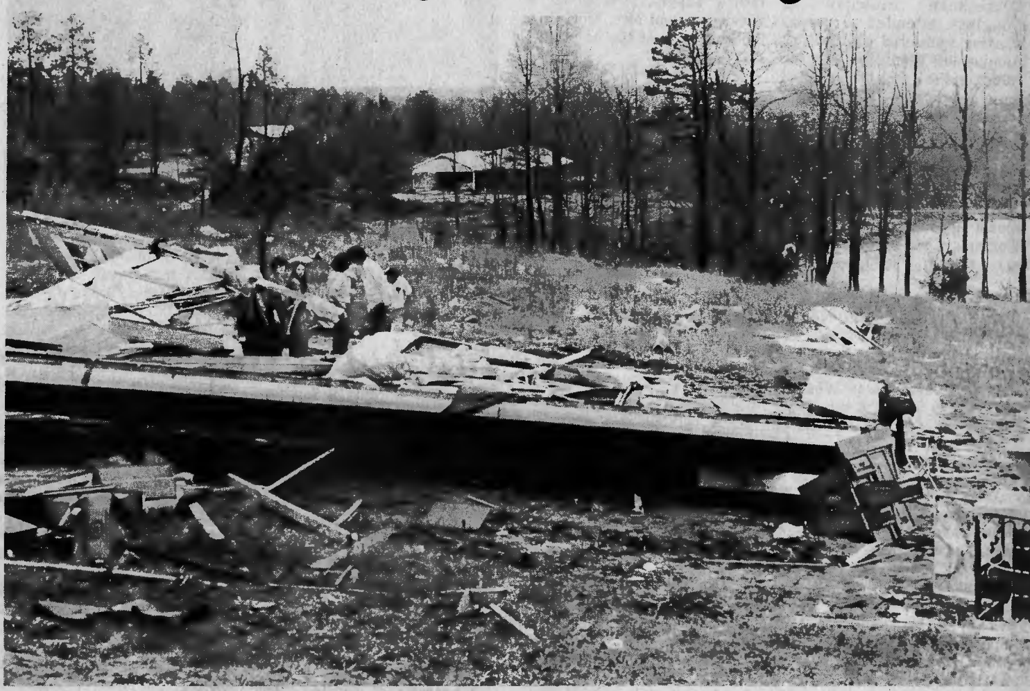
TORNADO DESTRUCTION — The mobile home of Mr. and Mrs. Clifton Southard was destroyed in the tornado which hit down near West End Monday afternoon. The family had fled to safety in a nearby
