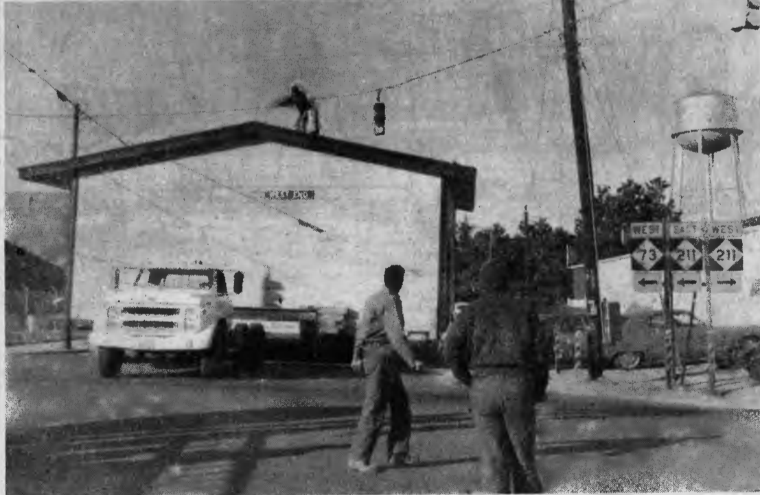
WEST END DEPOT MOVED — A telephone linesman rode atop the West End Depot, lifting traffic lights to clear space as the old landmark was moved through the intersection of highways in mid-town West End Tuesday morning. Clyde Auman purchased the depot from the Southern Railway and will use it for a warehouse and office at his peach orchard near West End. (Story Page 12-A).
