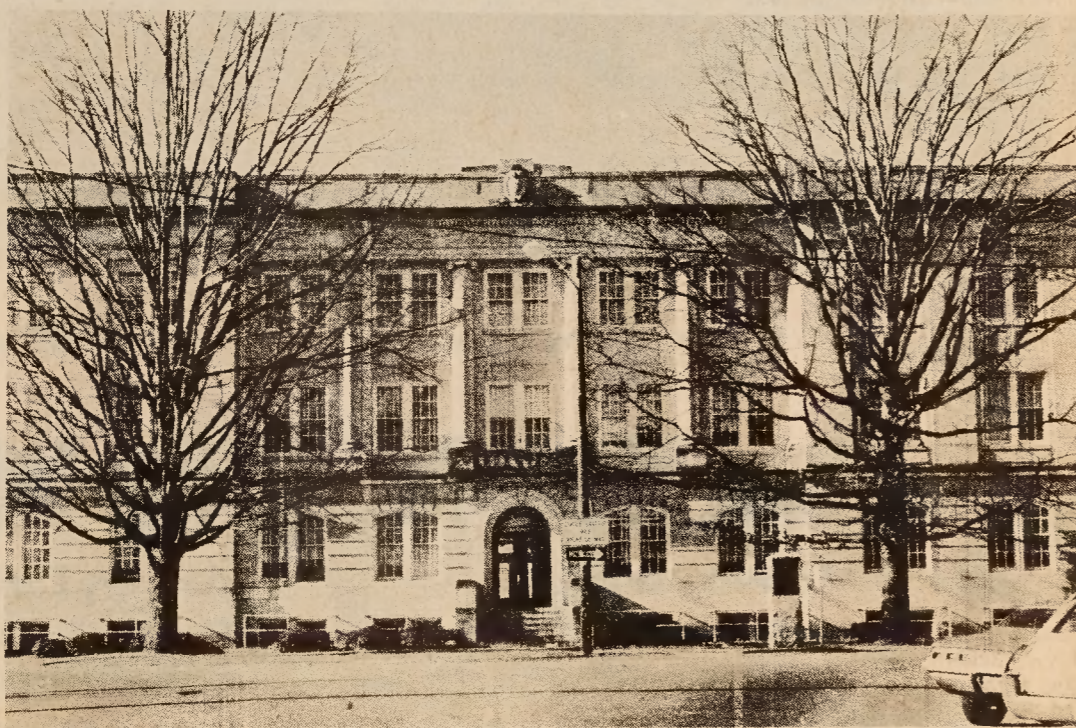
Moore County Courthouse was built in 1923.
