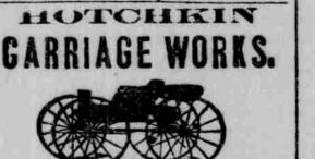
OUR No. 14 BUGGY. We manufacture Open and Top Bug-gies, consisting of the Side Spring, End Spring, Brewster, Timken and Edward Storm Spring.
