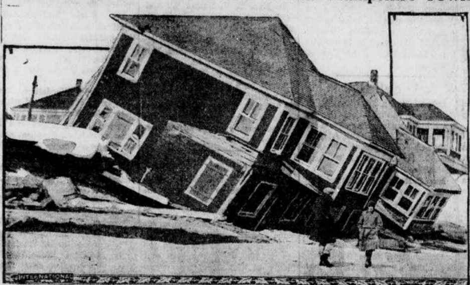
The great storms on the north Atlantic wrought havoc in some of the New England coast towns. This picture shows how houses in Hampton Beach, N. H., were wrecked when the heavy seas broke down the breakwater.
