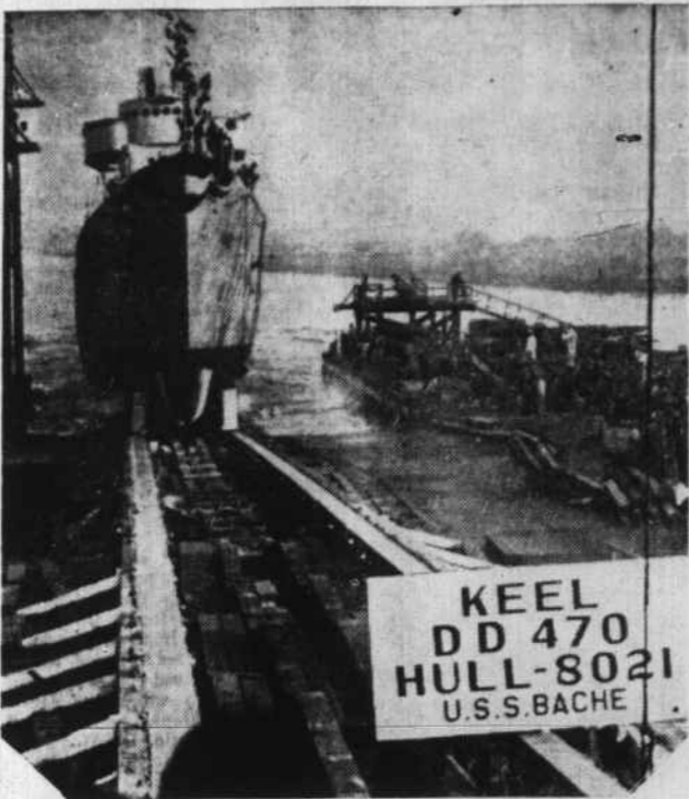
The destroyer Farenholt slides down the ways at the Staten Island, N. Y., yards of the Bethlehem Steel company's shipbuilding division. Men in the foreground are shown laying the keel of another warship, the destroyer Bache , in the space just vacated by the latest addition to America's navy.
