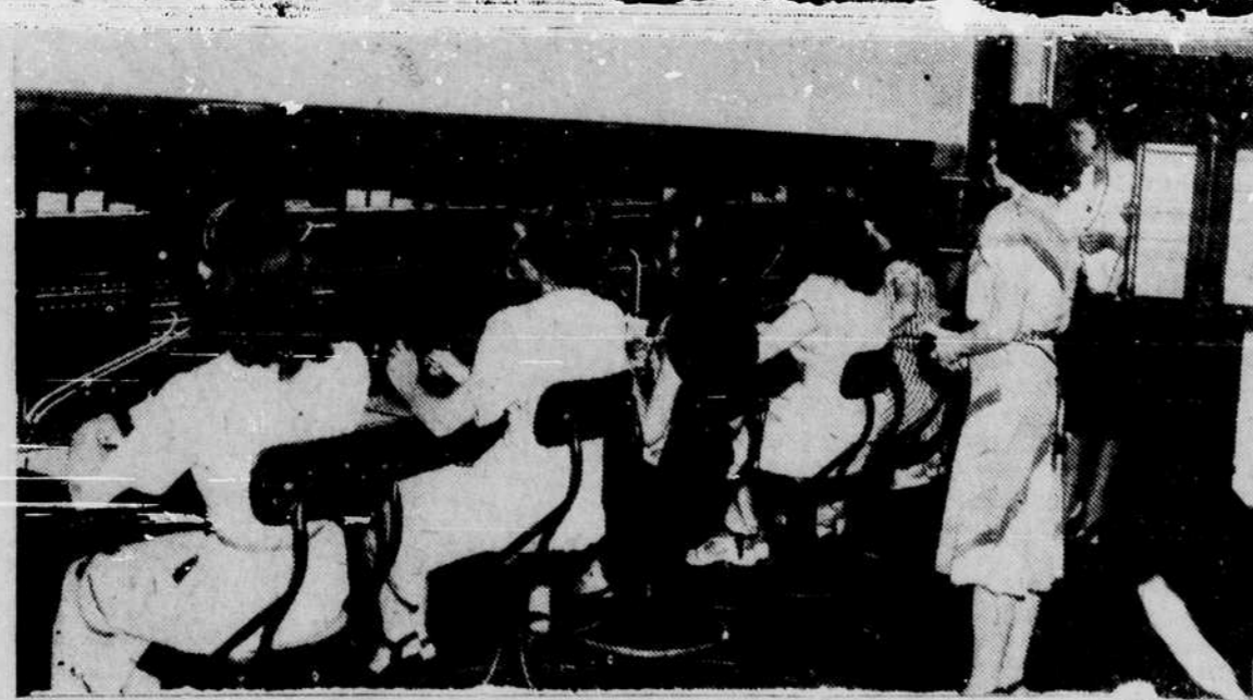
Promptly at 10:00 o'clock last Thursday evening, operators deserted the old switchboard in the local telephone exchange and took their seats at the new board where they are pictured handling their first long distance calls following the conversion from the manual to the dial system. Pictured above are (seated) Mrs. Thelma Caruso, Miss Dora Twiddy, Mrs. Anna Elizabeth Perry, Misses Dorothy Umphlett and B. Cherry; (standing) Miss Helen Stapleford and Mrs. Margaret Cone, supervisors.
