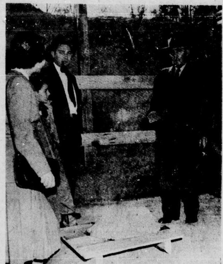
Mr. Van G. Taylor, one of the main benefactors, is pictured as he prepared to lay the first brick for Williamston's new 44-bed hospital the early part of last week.
