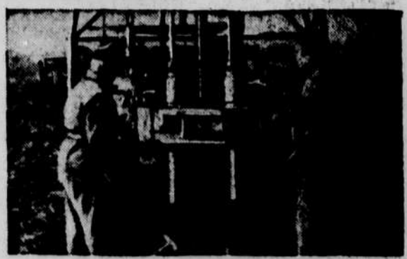
SHOT HOLE drilling machine is used by Sinclair to drill holes for explosive charges, the effects of which are recorded by sensitive Seismograph to map underground formations as deep as 15,000 feet.
