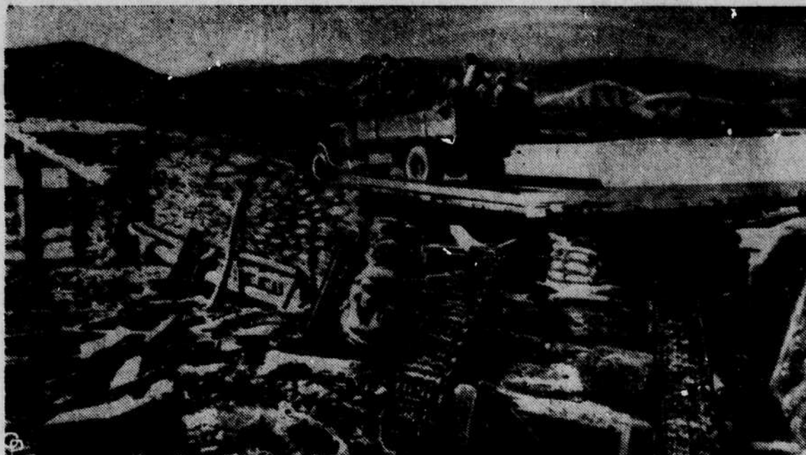
BRIDGEHEAD RESISTANCE by a Communist burned-out tank (lower, right) failed to halt a river crossing by troops of the Republic of Korea 8th Division at Yongju. Korean engineers patched up the bridge for oncoming units moving against the fast-faltering enemy. (United States Army Photo from International Soundphoto)
