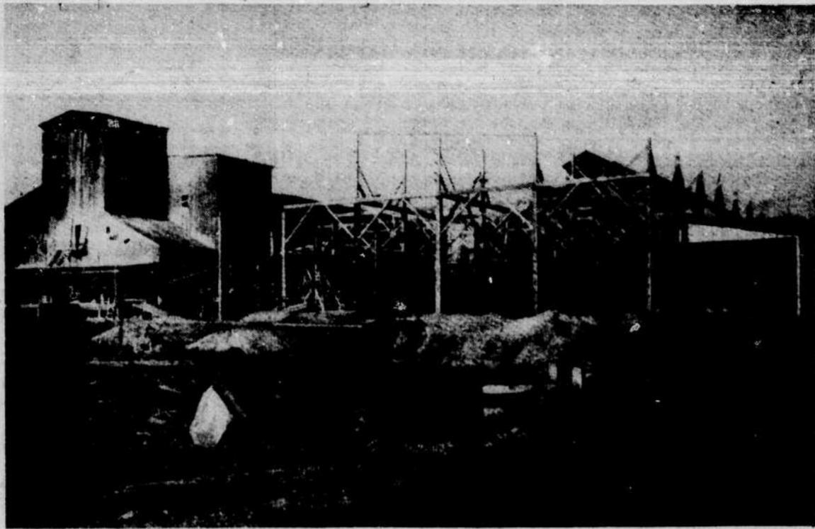
Despite unfavorable weather and other adverse factors, construction work continued to go forward on the addition to the plant of the Standard Fertilizer Division, Mathieson Chemical Company on Roanoke River here. The addition is a part of a quarter-million-dollar expansion and modernization program being handled by the company at its local plant.—Photo by Royal Studios.
