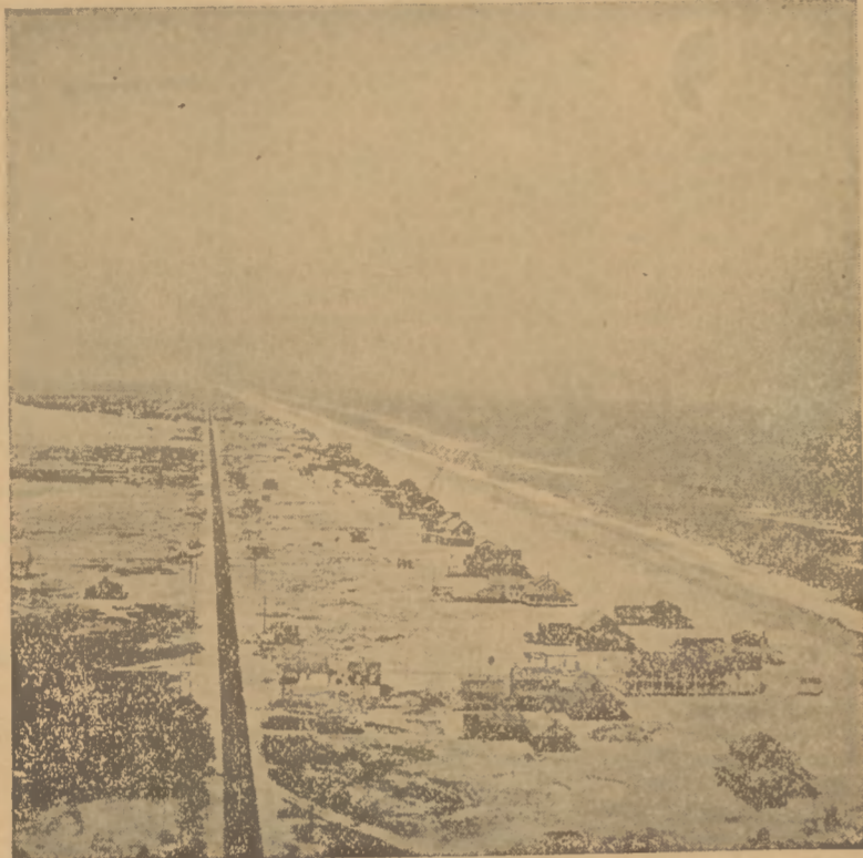
THIS AERIAL PHOTO, taken two years ago, shows the old Nags Head cottage line looking north from the Arlington Hotel.
