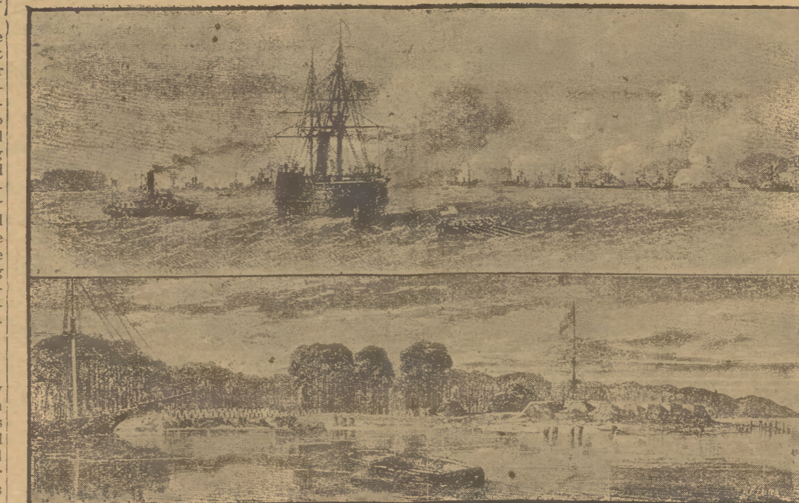
AN EYE WITNESS drew the above picture and it was sent to England and published in the London Illustrated News in March 1862. Roanoke Island people well remember the little hill that stood on the Battleground, and was known as the breast works. When the highway was cut through the island, the irrelevant men with scoops and mules, dragged the hill down to make a roadbed. The picture shows the 99th New York (Hawkins' Zouaves), and the 21st Massachusetts taking the Confederate fieldwork, on Roanoke Island at the point of the bayonet. This part of the battle was fought at the intersection of the road to Nags Head with the north and south road on Roanoke Island. Full details of this battle are published in The Times.
