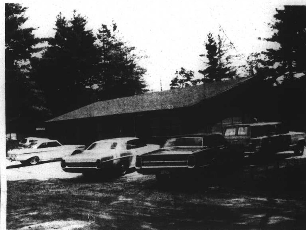
A view of the new U.S. Forest Service ranger's office on Smallwood Avenue in Highlands. (Staff photo by Helen Hopper)
