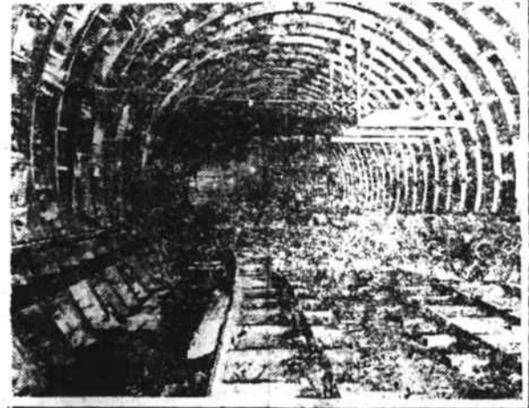
The great vehicular tunnel under the Hudson River at New York is rapidly nearing completion. This shows an excellent interior view of the gigantic engineering task.
