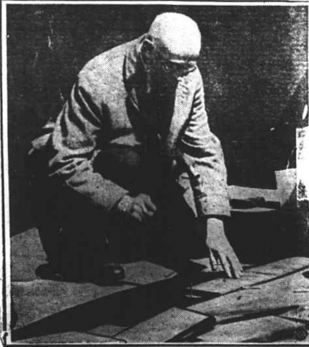
Rubber paving blocks, made from old auto tires, are being tried out in Boston streets. They are said to take the noise out of traffic and to wear better than many paving materials. John A. Rourke, a Boston city official, is shown laying the first blocks.
