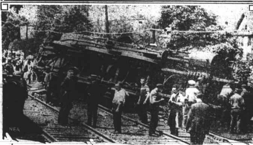
Four persons were killed and scores injured when a Jersey Central Philadelphia-New York express was derailed when it crashed into a ten-ton auto truck near Cranford, N. J. The engine and three cars plowed over the ties for a distance of three city blocks and then tumbled over.
