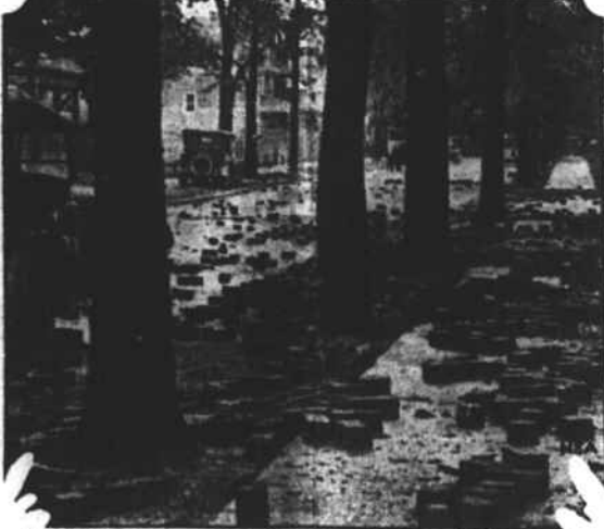
They had a heavy rain in Detroit—almost a cloudburst—and it flooded dozens of streets. Streets that were paved with wood or composition blocks suffered heavily, as the blocks floated away and were scattered all over the city when the water subsided.
