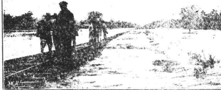
Eight and a half inches of rainfall in less than a week has caused a total loss of $1,000,000 worth of crops, food and traffic and it has paralyzed the Gulf States. The tracks of the Vicksburg, Shreveport & Pacific Railroad were flooded by the water, stopping all traffic for several days.
