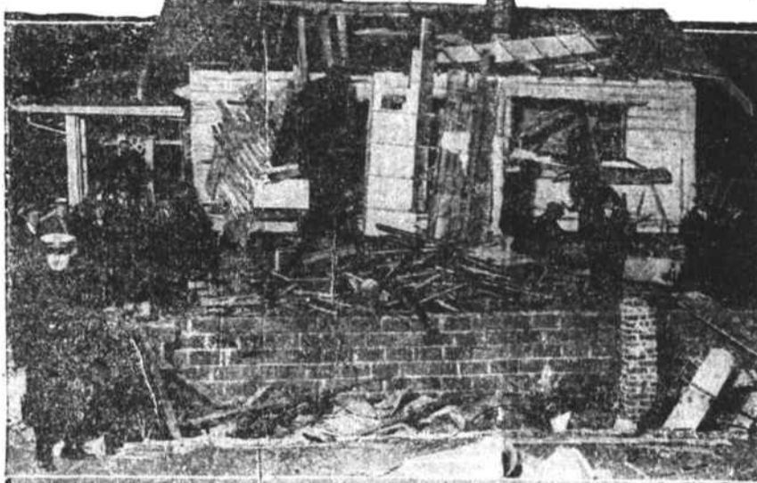
A brand new house was destroyed, two people were killed and five others hurt because someone accidentally trod on a match and touched off a gas explosion on Christmas afternoon at Topoka, Kan. The people were inspecting the house, which was unoccupied, and there was a leaky gas pipe. Photo shows the ruins, with the damaged wall of a neighbor's house in the background.
