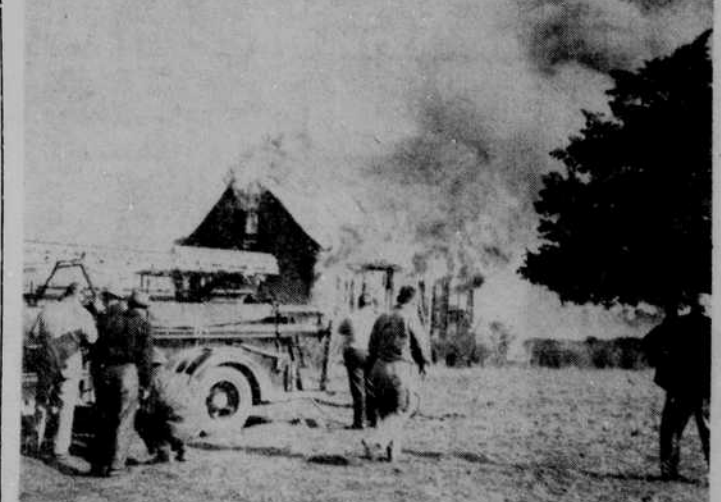
Plymouth firemen were unable to do much about this fire, which destroyed the home of Annie Johnson, colored, on the Mackeys Road near here last week. An overheated oil heater caused the blaze, which completely destroyed the house and its contents. There was no insurance.—Polaroid 1-Minute photo by Henry Cannon.
