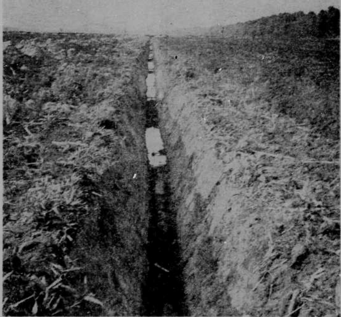
The above photo shows a drainage ditch on the D. M. Roberston farm in the Lake Phelps area and is only one of many such ditches which have been dug during the past year in this county and adjoining ones. H. E. Newland, of the Soil Conservation Service, reports that great progress was made in the county last year in solving drainage problems with the use of draglines. As many as 13 such machines have operated at a time in the county during the year.—Photo by Newland.
