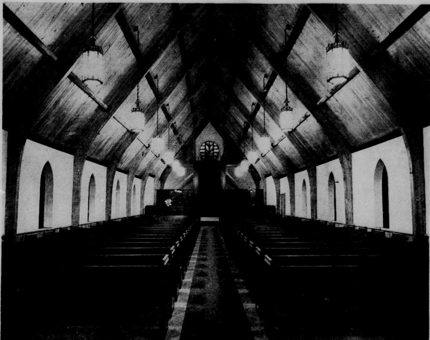
SANCTUARY: This picture shows the forward part of the new First Christian Church of Plymouth, which has now been in use for a little over a month. Finished in natural wood colors, the slanting ceiling and massive laminated trusses of Oregon redwood make the interior one of the most beautiful in this part of the state.
