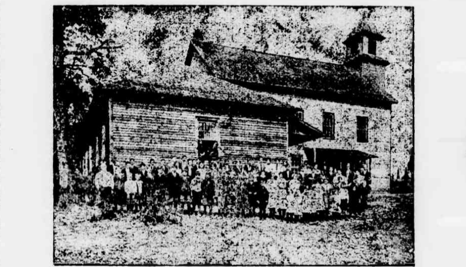
This is where the new superintendent of the county schools has seen three years of good service. This building will be displaced by a modern $1250 brick structure.
