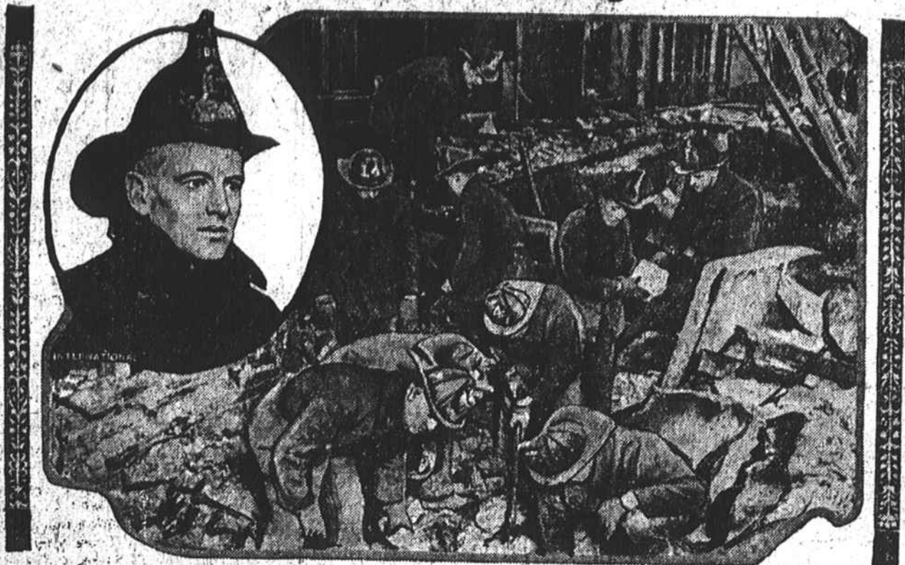
At least seven firemen and one civilian were killed and a score were injured in Chicago when an explosion in a burning building caused a wall to fall, burying the men. Above are seen firemen searching for the bodies of their comrades, and Father Ed A. Jones, who made his way into the ruins to administer the last rites of the church to the dying.
