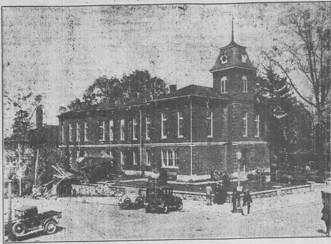
Picture shows big trees blown down on Court House Lawn in wind storm last Thursday. The bandstand was demolished, as can be seen, while two large trees were uprooted just to the right of the entrance. This picture was taken by M. D. Foxman soon after the storm abated, and shows power of the winds.
