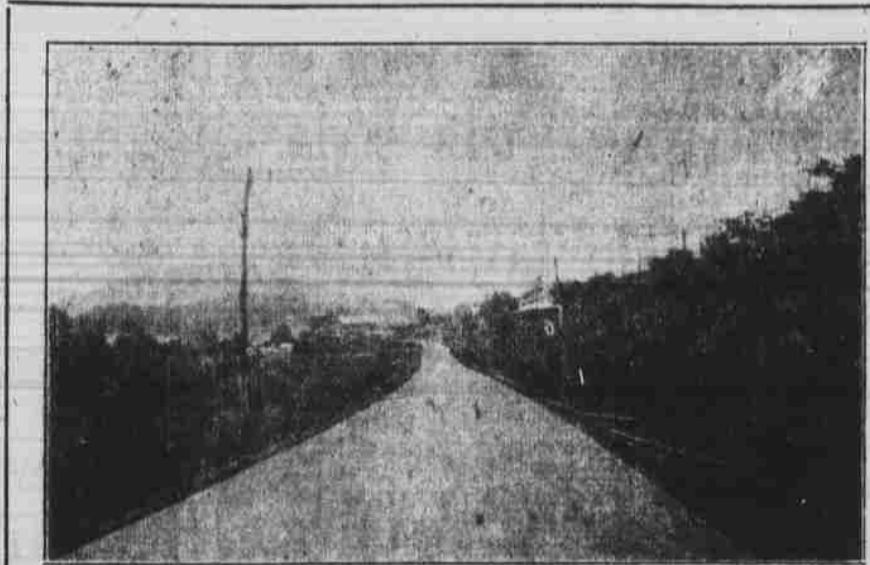
View of Macon County's Link of Atlanta-Franklin-Asheville Highway.
