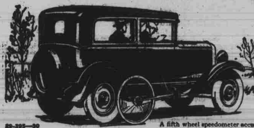
A fifth wheel speedometer accurately measures speed and mileage on all Chevrolet test runs at the Proving Ground.
