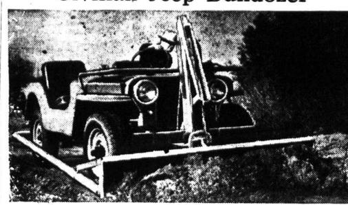
special TMC Hydraulic lift that raises and lowers over blade, all four wheels are driving as this civilian jeep errapes roads or fills ditches, jobs it does as easily as pulling plows or powering farm machinery through a power take-off. Shifted to two-wheel drive, the Willys-Overland vehicle races to the next task at speeds up to 60 miles an hour.
