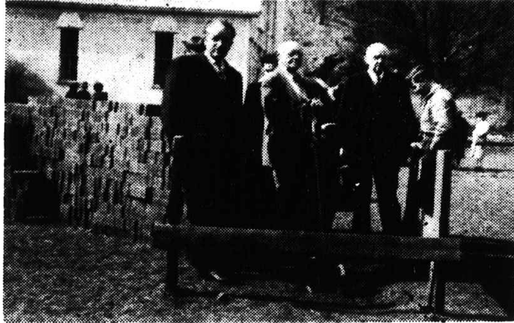
Scene At Ground Breaking At Scotts Creek
