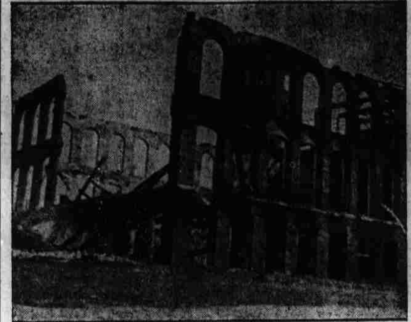
What was left of the Textile Building of A. & M. College at Raleigh which burned recently. The contract has been let for its construction on a larger scale to be completed by August 1st, and manufacturers of textile machinery are being invited to again donate machinery for its equipment. The equipment for the burned building was donated in this way in 1901.
