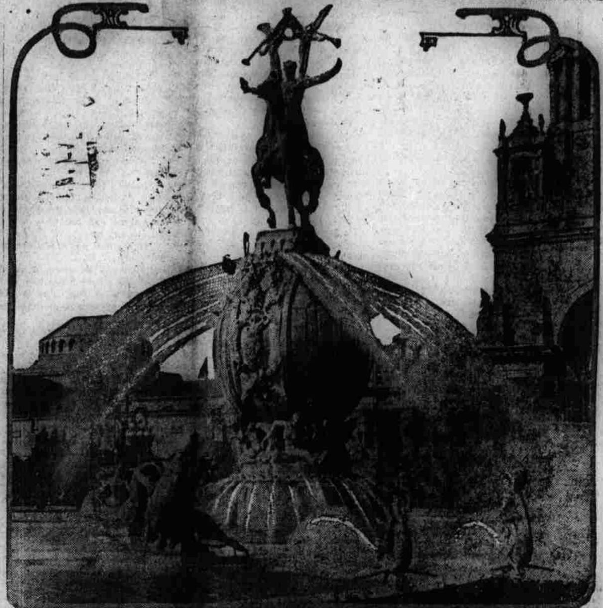
The labor that went into the building of the Panama canal is symbolized in the Fountain of Energy, by A. Stirling Calder. This heroic sculpture stands in the center lagoon of the three lagoons of the South Gardens and faces the main entrance gates. The waters were first released on opening day, February 20, coincidentally with the opening of the portals of the exhibit palaces and by the same means: the electric spark transmitted across the continent when President Woodrow Wilson opened the great exposition at San Francisco by wireless.
