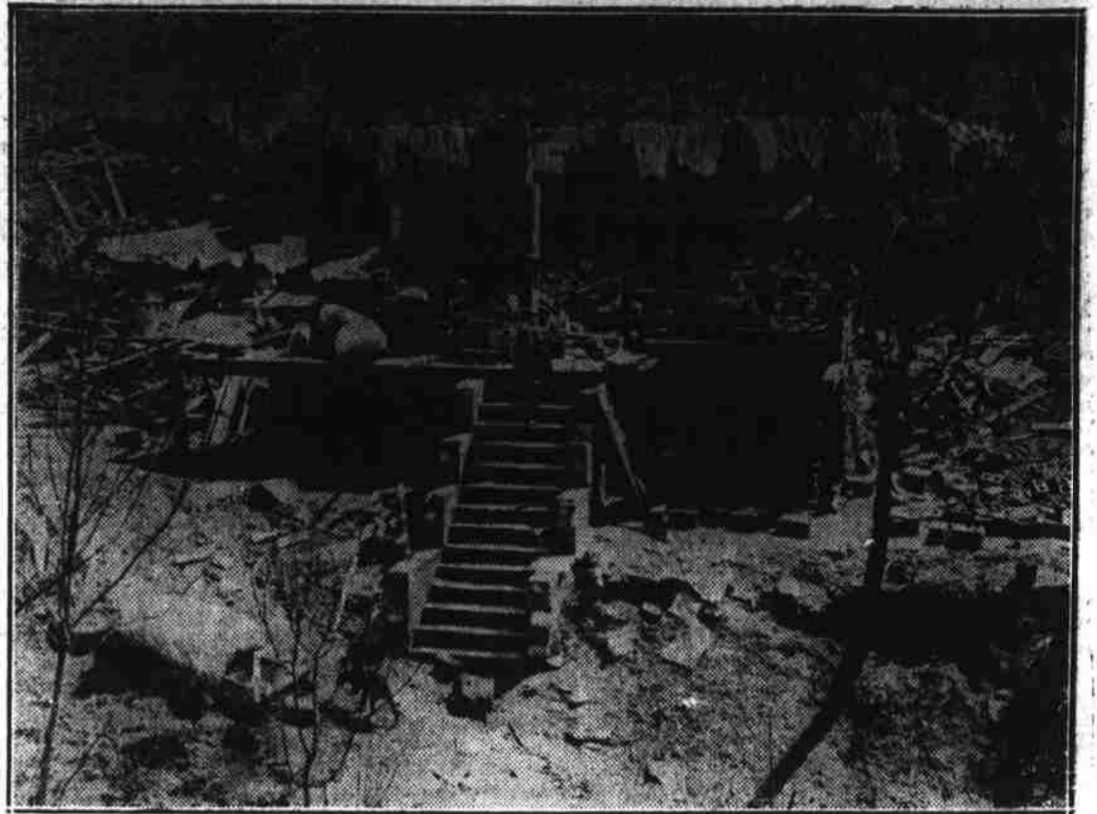
Remains of mountain homes, such as this, were left by the wind storm which swept through a section of Madison county late Monday afternoon. The photo shows what is left of the one-story cement block house that belonged to Mr. and Mrs. Lyda J. Brown on Shoal Hill road in Little Pine Creek section. The wind forced the walls outward, thereby saving its occupants from serious injury. Mrs. Brown's leg was injured and her daughter, Gracie, suffered an injury to her arm.
