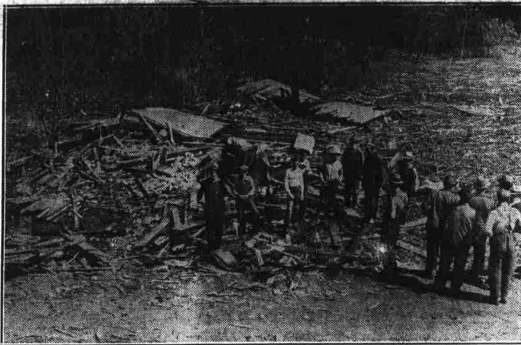
The destruction of the house, the remains of which are shown here, caused the death of its owner, A. F. Sluder, 63-year-old farmer of the Little Pine Creek section. The wind picked up the three-room house, which was on a knoll, carried it across the road, and deposited it in a field. As the house settled, it fell apart. Sluder's skull was crushed and he died Monday night.
