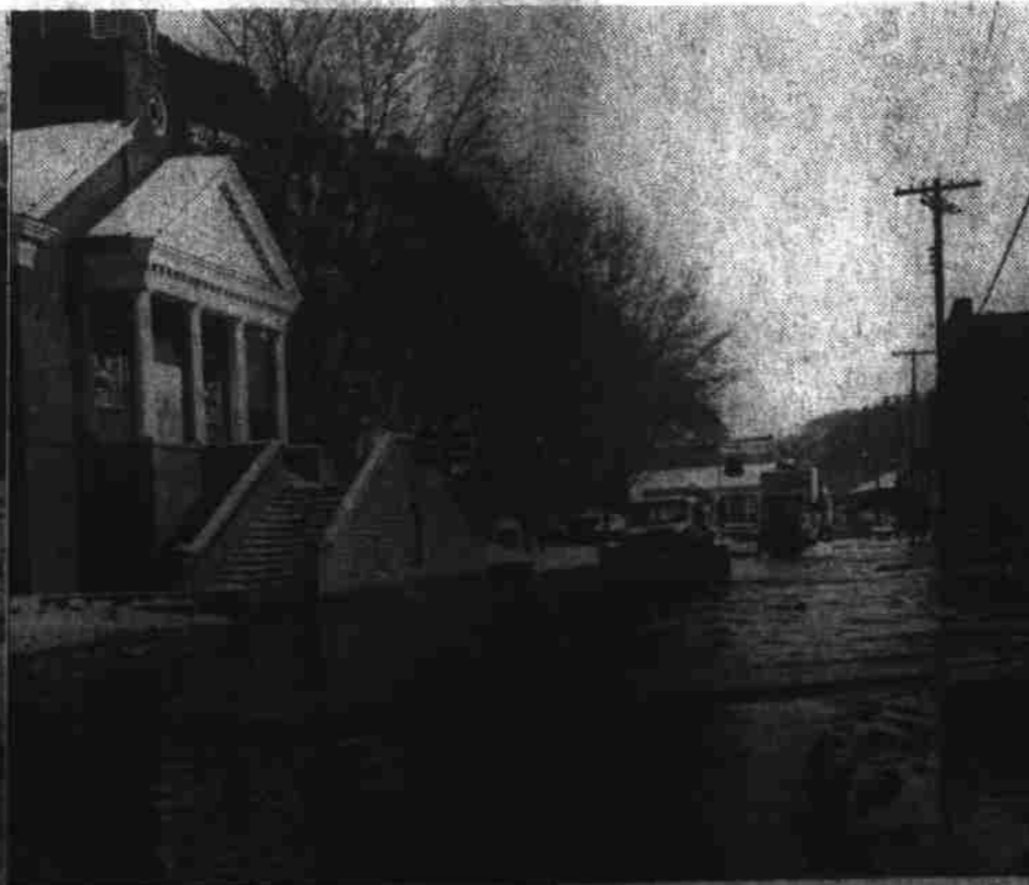
Spur bridge (at right in photo) serves Marshall High School on Blannhasset Island. Presence of this ice pack on downstream side of Marshall caused storm sewers to back water into business district (center), with depths up to three feet. View looks toward Asheville. Water in front of Presbyterian Church between two and three feet deep. Meanwhile, on
