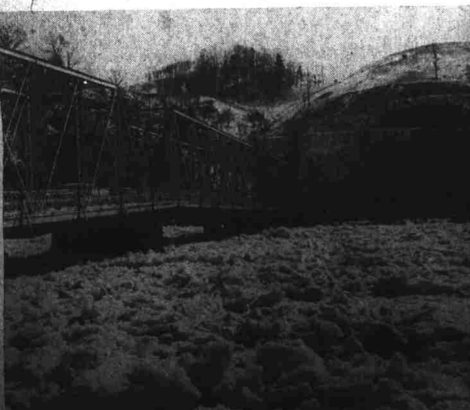
LIKE ARCTIC WASTELAND, frozen French Broad River at Marshall this week was threatening and treacherous. As river froze nearly solidly across, pressure mounted against old Asheville Highway Bridge (left) which crosses river from center of town opposite the Courthouse to Bailey's Branch Road which goes through Sandy Mush to Asheville.
