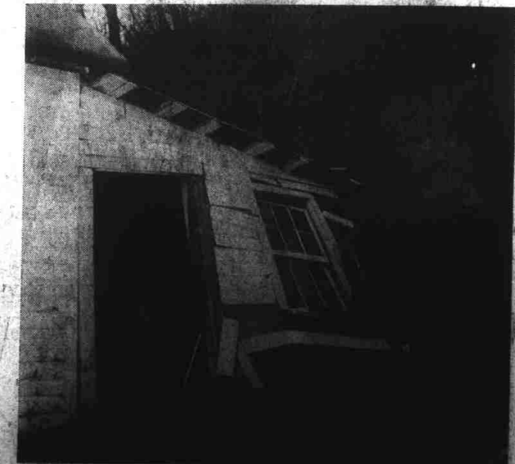
ONE OF THE HUGE LANDSLIDES IN Marshall Friday, after torrential rains Thursday night, crashed through the home of Mr. and Mrs. Evan Worley on a street behind Blannahammett Island. Tons of dirt poured into the kitchen (above). The right side of the house was torn loose from the foundation. The Worleys were uninjured. The second slide covered Hill Street with more than six feet of earth, endangering the home of Mr. and Mrs. James Penland.
