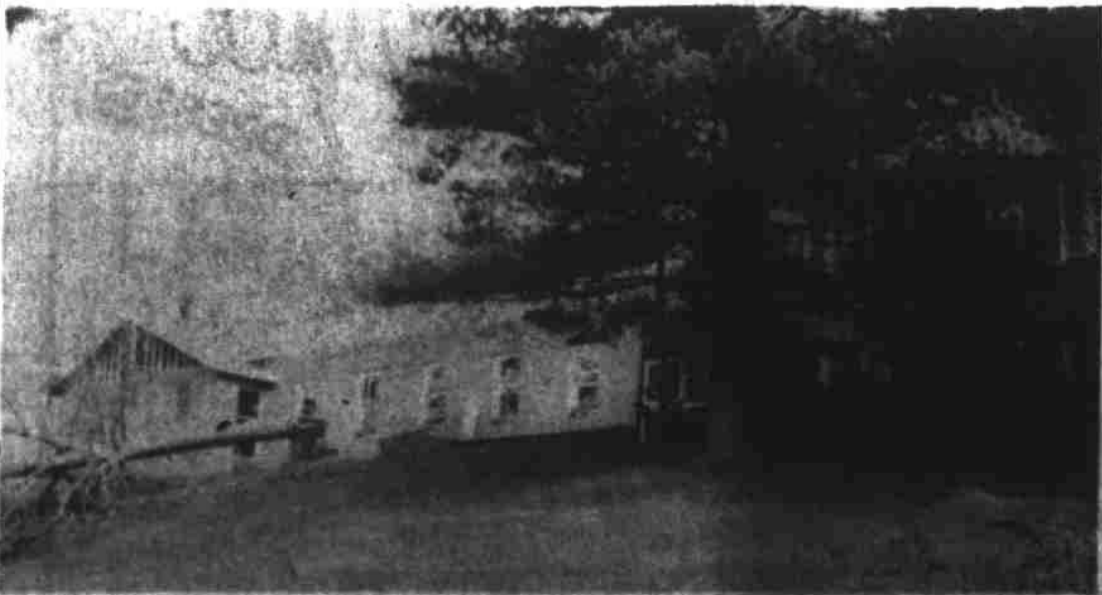
Pictured above is the new Madison Seminary Baptist Church now under construction. Behind the large tree is the present church which was built in 1925. The old structure will be removed when the new church is completed. The new building is being constructed under the supervision of the Slagle brothers. The building committee is composed of Lloyd Slagle, Charles Crowe and Talnage McLean. The building started last Fall, is expected to be completed in the Spring.
