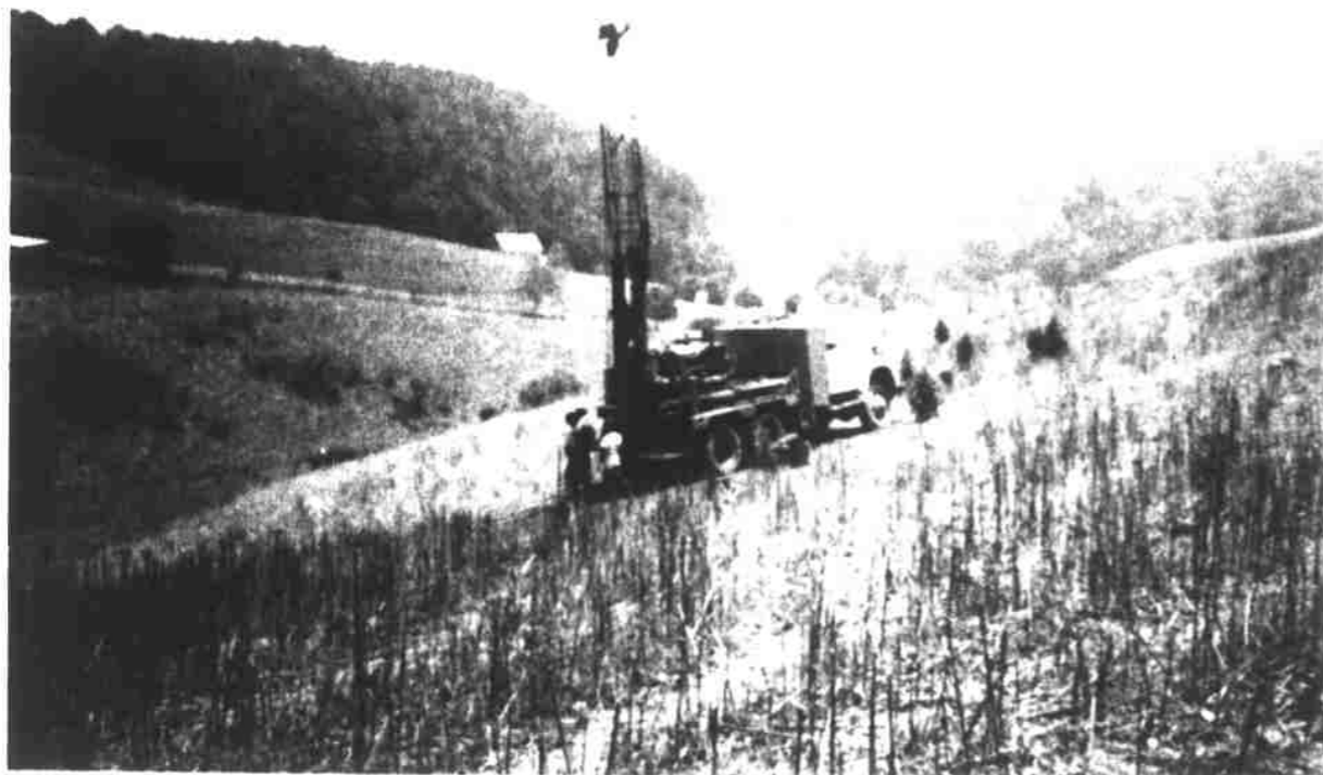
AN UNUSUAL VIEW from the site of the proposed new consolidated high school for Madison County shows the start of core drilling Monday morning by Law Engineering Testing Company of Charlotte. In
