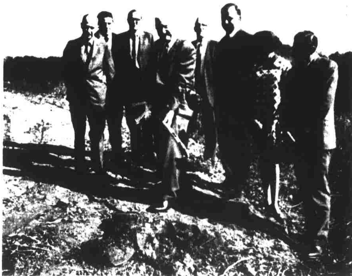
OFFICIAL GROUNDBREAKING for the Madison County Consolidated High School, located on a 57 acre site adjacent to the Marshall By-Pass and Walnut Creek Road, was held Wednesday afternoon. Grading has started and plans are to let the general contract for construction in December or January, and to have the complex of buildings ready for use in the fall of 1973. Pictured above taking part at the ceremony, left to right, Emery Wallin, Bobby Ponder members of the board of education; R. L. Edwards, superintendent; holding spade is Ralph M. Lee, member of board of education; William C. Reeves, board attorney; J. Bertram King, of Asheville; architect; Mrs. Bobby Jean Peek Rice member of board of education; and William M. Roberts, chairman of the board of education.
