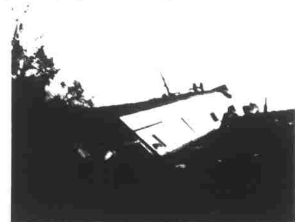
PICTURED ABOVE is the mobile home of Mr. and Mrs. Jackie Roberts of the Anderson Branch section, which was destroyed by wind on January 25.
