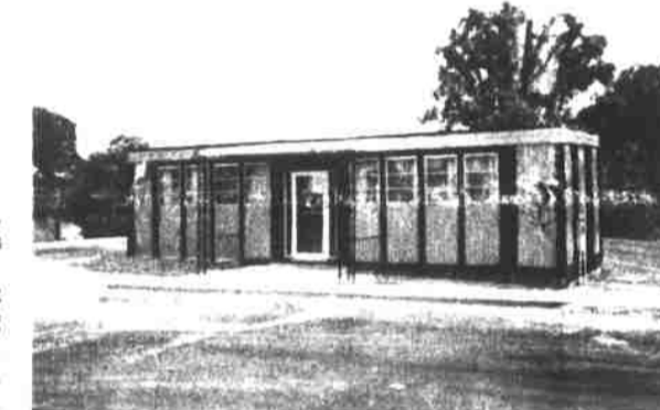
SHOWN ABOVE IS the new Citizens Bank Drive-In Office which will open this Saturday at Mars Hill. The convenient structure is located at the corner of Cherry and Anderson Streets across from the Community Medical Center. More details are published in an advertisement elsewhere in this issue.
