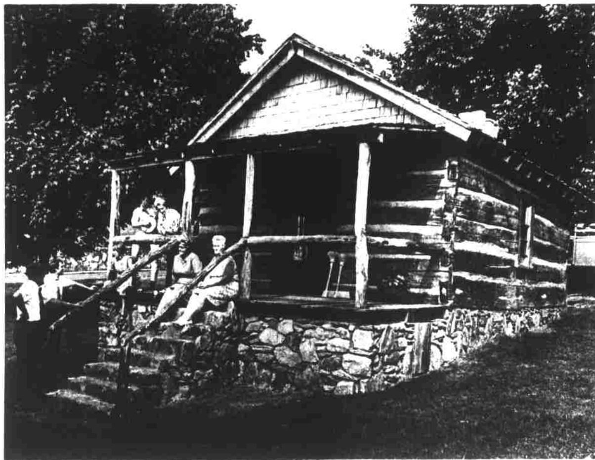
A CENTURY-OLD LOG CABIN on the campus of Mars Hill College was restored this year for use as The County Boutique, the outlet for Madison County Crafts, a cooperative program which involves some 150 people in Madison and rural Buncombe counties. The log cabin was the old Frog Level schoolhouse, according to Dr. John McLeod, college historian, who called the building "the last existent field school in the nation." After the post-Reconstruction era
