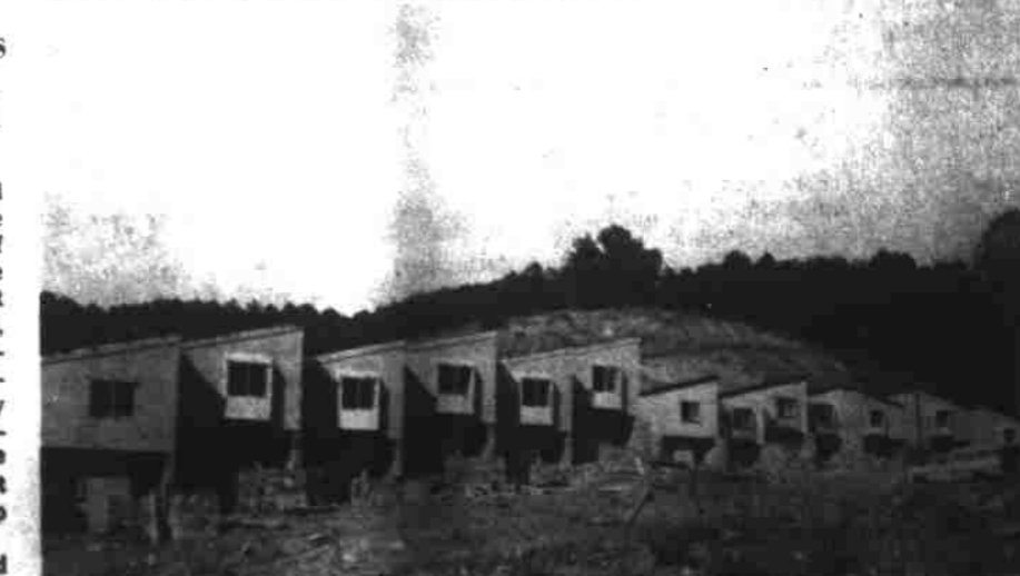
ONE STEP NEARER completion is the low-rent housing project located on Walnut Creek Road in Marshall. Buildings on the other three sites are also being completed and are expected to be finished later this fall.
