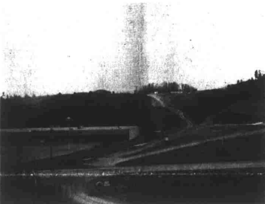
ANOTHER ADDITION JUST OFF THE Marshall by-pass is a new road under construction from the shopping center to the county school bus garage and to Mato, shown above. On right is the Farm Credit Bureau building.
