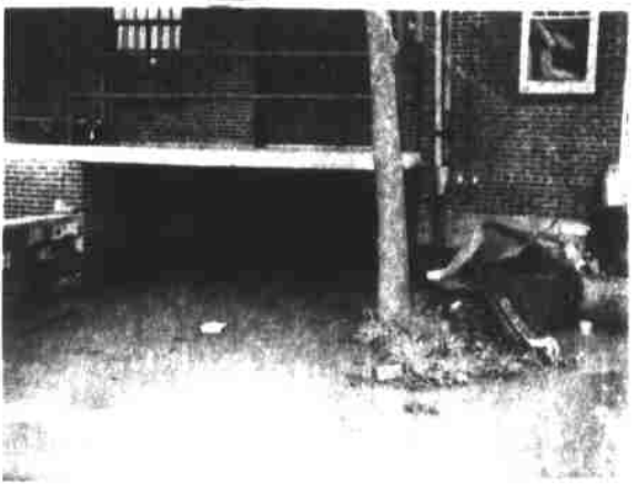
BASEMENT OF MARSHALL POSTOFFICE FLOODED. Picture taken Saturday morning after water receded a foot. Back Street was closed Friday night due to flood conditions. Other basements flooded similar to above.
