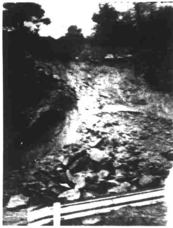
HUGE CAVE-IN on Roberts Hill Road early Saturday morning sent tons of rock and dirt across Highway 25-70 just north of Main Street.
