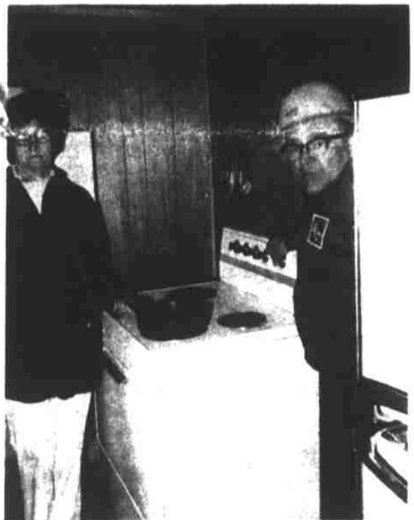
MR. AND MRS. COLLIE PAYNE, of the Big Pine section, are grateful to French Broad EMC personnel for changing transformer and wiring last week from 120 volts to 240 volts so they could use a recently purchased electric range in their mountainous home. This was achieved by using "Berry", their 6-year-old steer to pull the steep grade for about one-third of a mile with transformer, equipment and wire on a sled. Top photo shows Collie looking at loaded sled starting up the mountain. Center picture shows left to right, "Sambo" Waldroup, Ivan Bradley, Collie Payne and J. C. Brazil watching "Berry" do his thing. Bottom photo shows Mrs. Payne and "Sambo" Waldroup in Payne kitchen with new range. Waldroup and Brazil are servicemen for the co-op; Bradley is co-op Work Order Accountant. Arnold Garrison, warehouseman, was the photographer.
