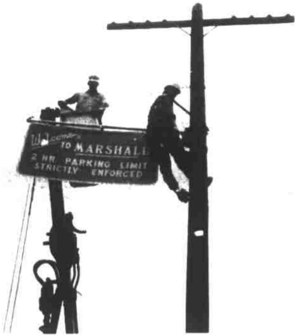
PICTURED ABOVE is one of three signs installed in Marshall last week. Shown installing the sign at the lower end of Main Street are Ray Caldwell, left, and Randy Roberts, right, French Broad EMC linesmen. Other like signs are at the upper end of Main Street and on Lower Bridge Street. The wording speaks for itself. The new two-hour parking system will begin here this Friday.
