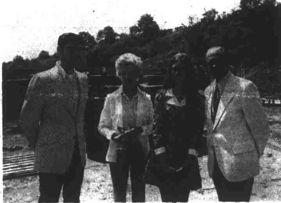
INSPECT NEW DERINGER PLANT SITE — Pictured above are four officials of Deringer Mfg. Co., viewing the progress being made on the new Deringer plant on the industrial site on the Marshall bypass Monday. Left to right, Pat Clemens, local plant manager; Mrs. Evelyn Deringer of California, widow of the late Paul Deringer, founder of the huge electrical contacts plant; Miss Jean Clemens, secretary at the Marshall plant; and Porter Duell, of Libertyville, Ill., executive vice-president of Deringer Mfg. Co.
