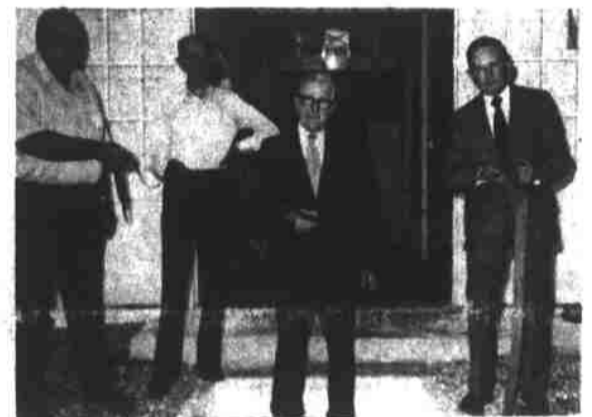
MAYOR PONDER cut ribbon while standing in newly constructed "foot rinsing" pool at entrance to dressing rooms. Others in picture, l to r, Alderman Crowe, Alderman Wild, Alderman Penland.
