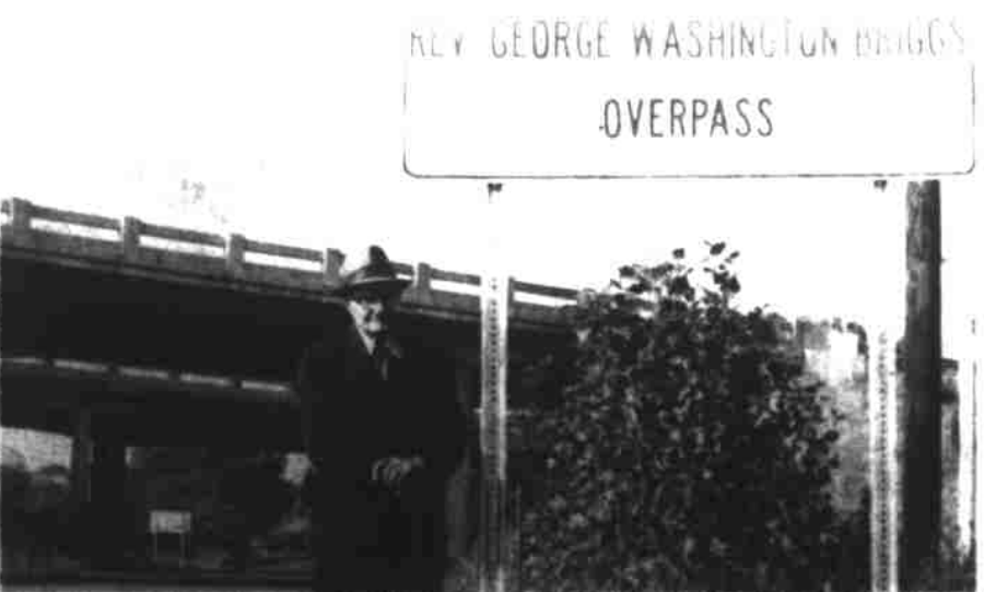
THE 1-46 overpass at Chestnut Grove, Tennessee has been named in honor of a prominent minister and farmer whose home was taken for the highway right of way. George Washington Briggs 94, who moved from Madison County, North Carolina in 1937 to Jefferson County, Tennessee has pastored Free Will Baptist Churches throughout Madison County and Western North Carolina for a number of years. He was one of the founders of Brown's Chapel Missionary Baptist Church located in the Chestnut Grove Community in Tennessee. Mr. Briggs now resides in Madison County part of the time. He is the father of nine children, namely Roscoe Briggs, Carrie Briggs Fisher, Myrtle Briggs Fisher, Queen Briggs Edmonds, and Cora Briggs Hunter all of Madison County. Hubert Briggs, Carl Briggs, Charles Briggs and Dorothy Briggs Sellars all of Tennessee. The Briggs' are one of the oldest most prominent families in Madison County.
